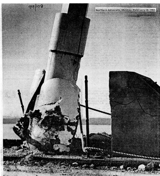
Figure 15: The base of the flagstaff after the 1983 explosion, Northern Advocate. Monday, February 28, 1983
